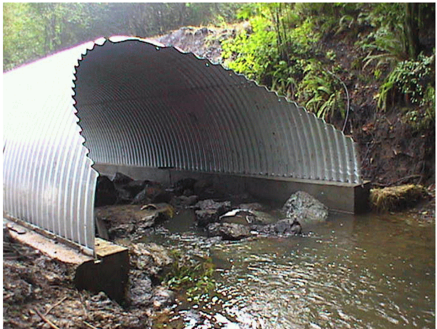
Photo of a multi plate arch culvert being fabricated on concrete footings
