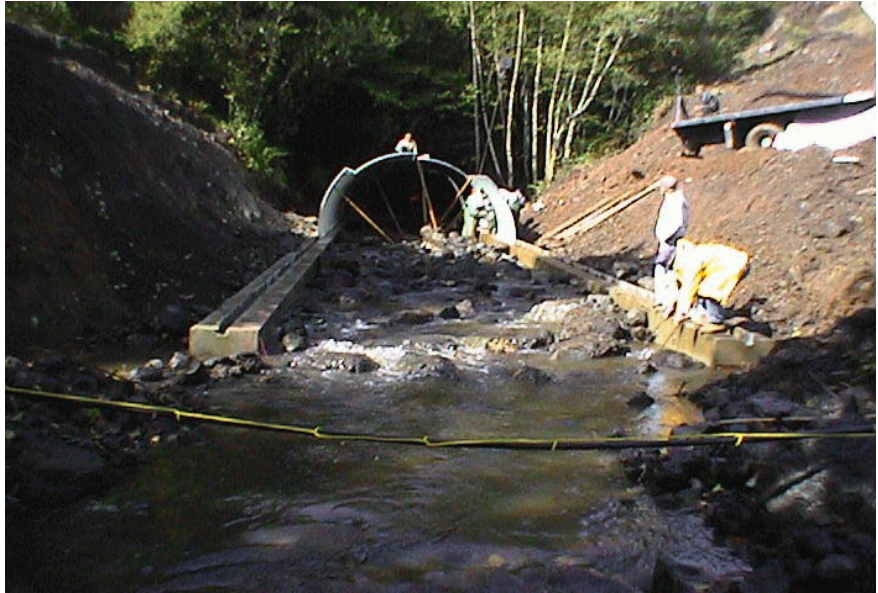
Photo of a multi plate arch culvert being fabricated on concrete footings
